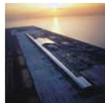
Kansai International Airport Passenger Terminal Building Osaka, Giappone
