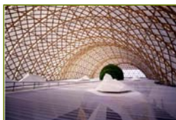
Japan Pavilion for Expo 2000 Hannover. Shigeru Ban architecte.
